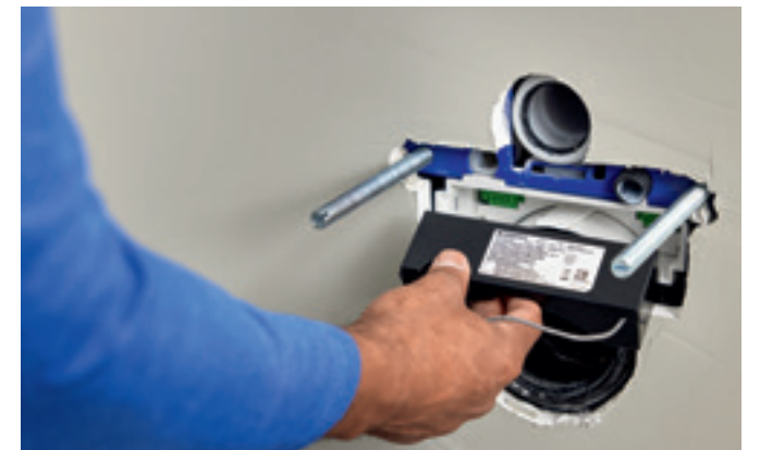
Installation of the GEBUS converter for WC controls with integrated power supply unit
