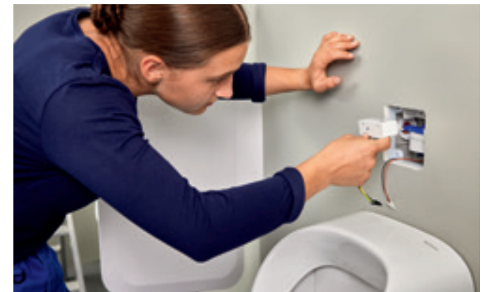
Installation of the GEBUS converter for urinals, concealed urinal controls and washbasin taps
